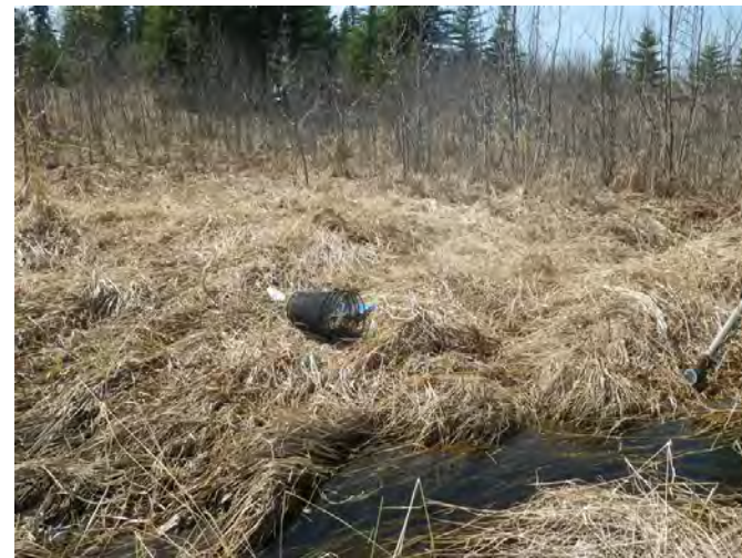
View downstream through centre of the proposed pipeline corridor (09-05-13).
