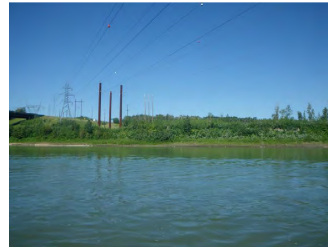
View of left bank approach at centre of the proposed pipeline corridor (29-07-14).
