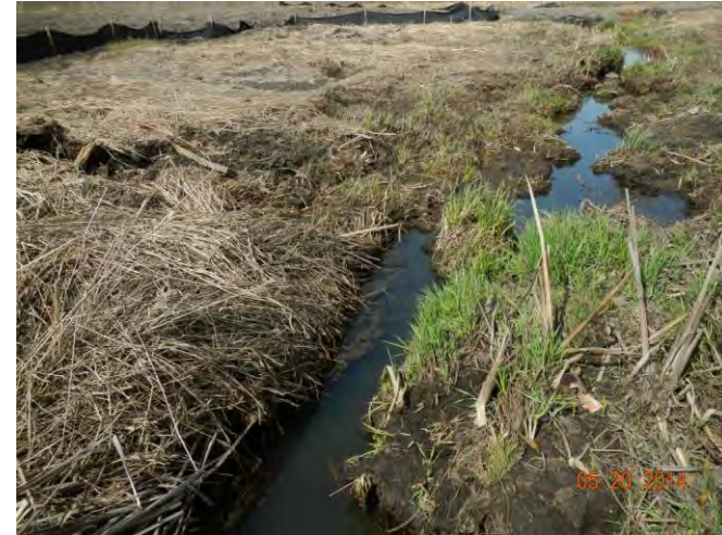
View downstream through centre of the proposed pipeline corridor (20-05-14).
