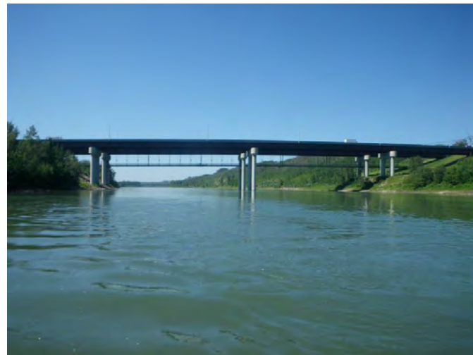
View upstream through the centre of the proposed pipeline corridor (29-07-14).
