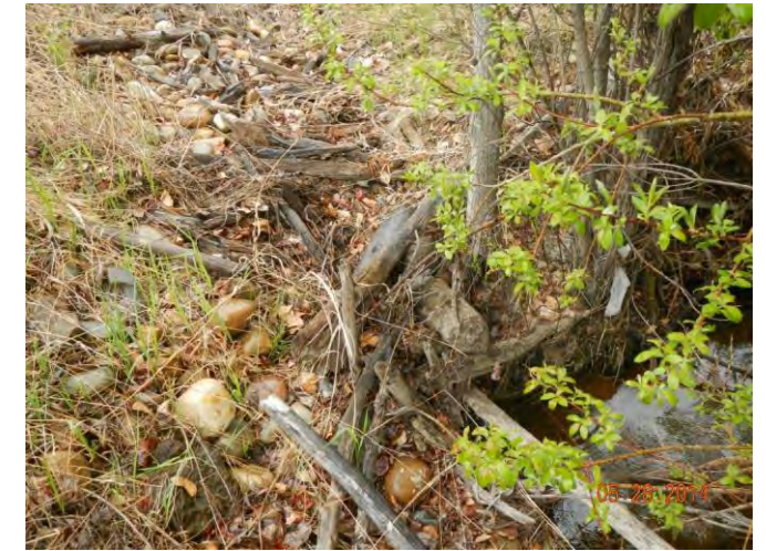
View of right bank approach at centre of the proposed pipeline corridor (28-05-14).
