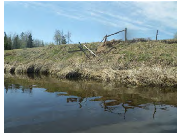
View of left bank approach at centre of the proposed pipeline corridor (10-05-13).
